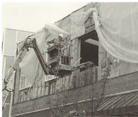
Construction underway at our Hillsboro, location, 1001 SW Baseline Street.
