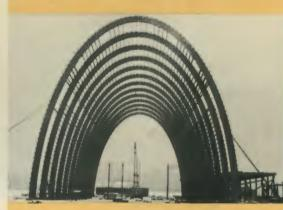
Wood engineering produces spectacular results. The Radar Test Laboratory, Dayton, Ohio, used glued-laminated Douglas fir lumber for stability and permanence.
