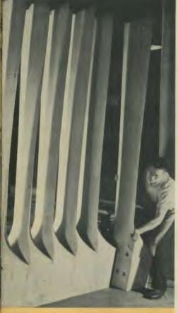
Sitka spruce is a unique wood with a multitude of specialized uses. It is used for propellers in all large wind tunnels and provides virtually all piano sounding boards produced in this country.
