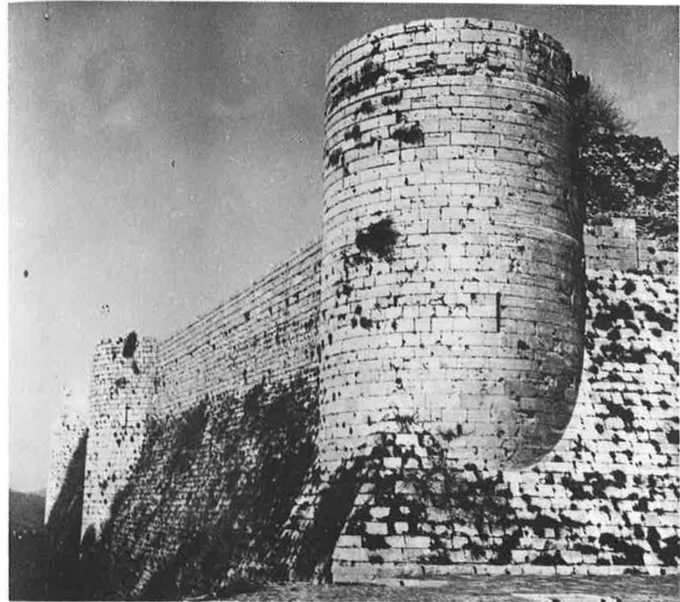
Fig. 12 Inner wall, Western front.
