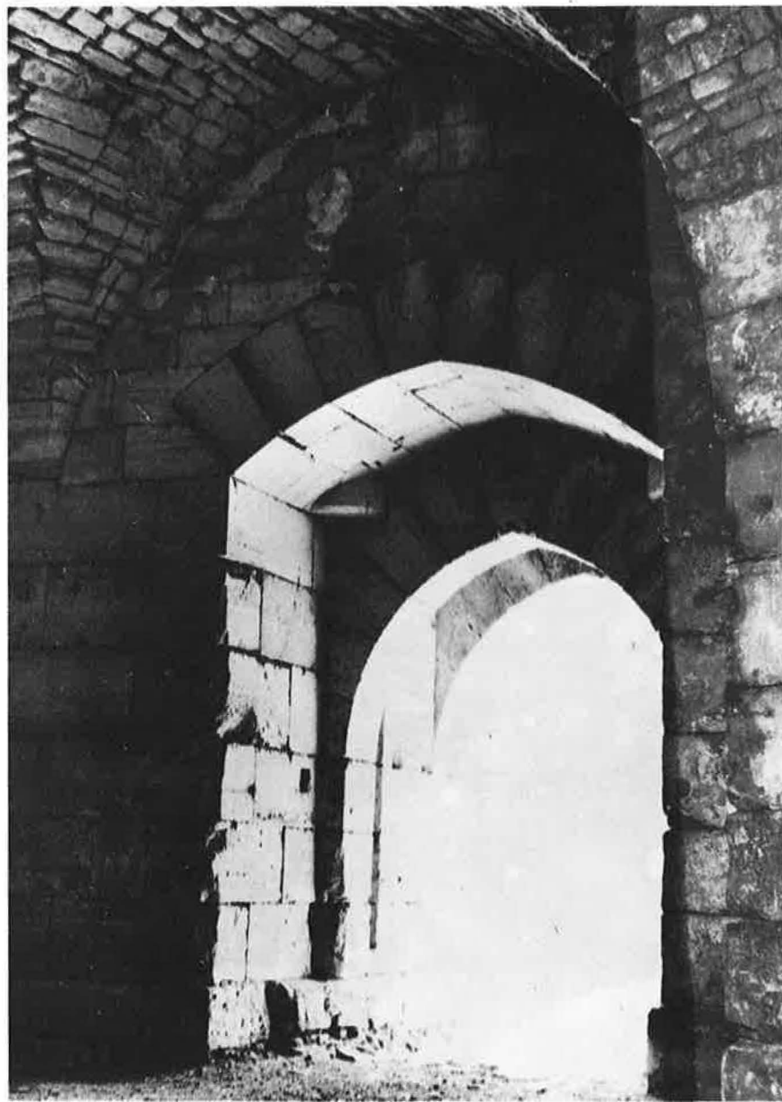
Fig. 7 Door of Tower No 9 Seen from inside.
