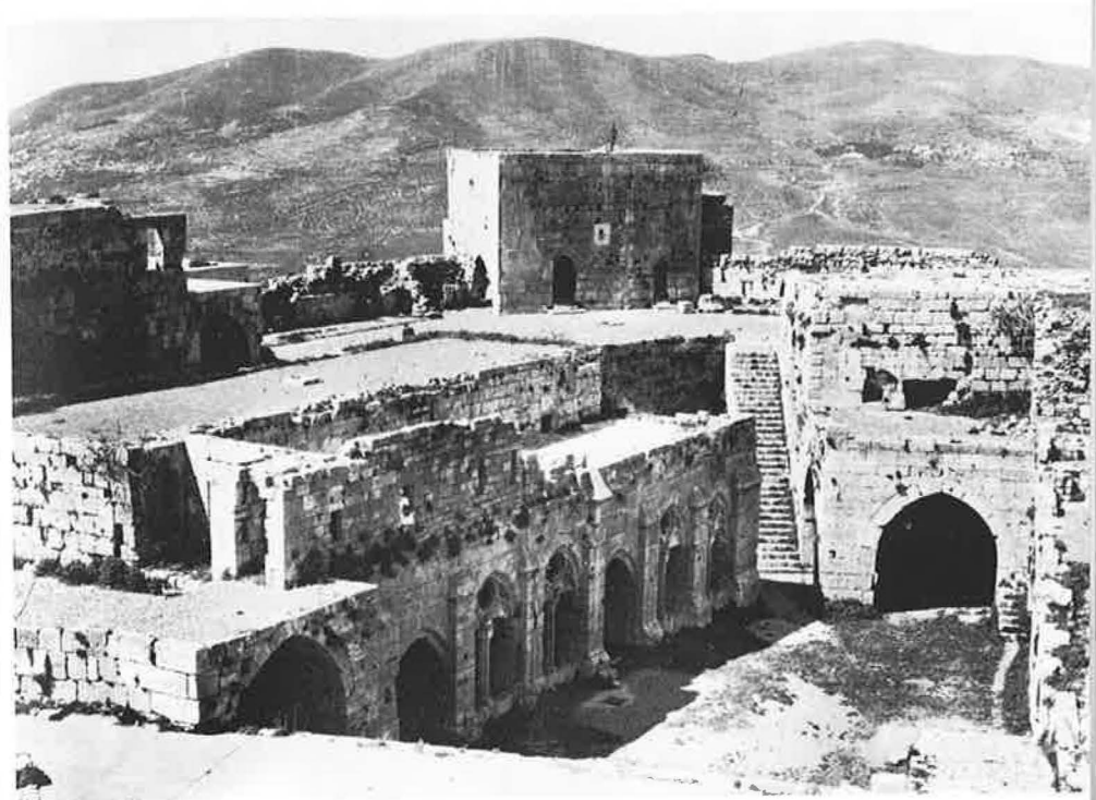
Fig. 15 Tower N° 16 and Façade of the Corridor.
