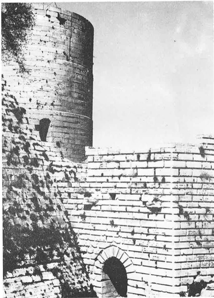
Fig. 8 Tower N° 9 and the south-East corner tower of the upper level
