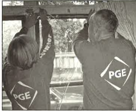
PGE volunteers weatherize a window for a Community Action client.
