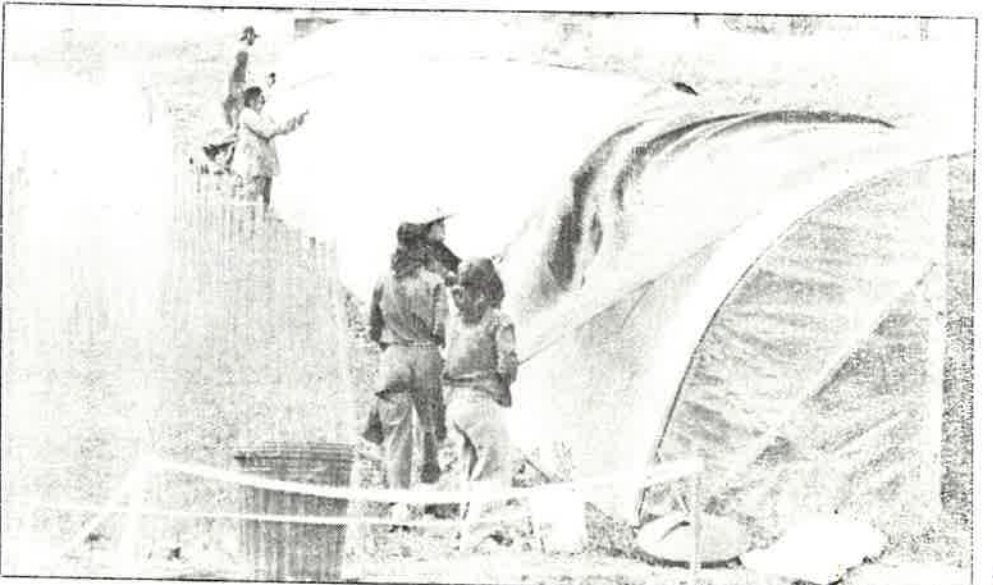
Greenhouses, like these built last year, are still part of the Rajneesh idea. They even grow bananas. But the scope of Rajneeshpuram has outgrown the "simple farm" concept by leaps and bounds. A 500-unit hotel is in the planning stages, along with an industrial park, factories for light manufacturing, and an adult education center.
